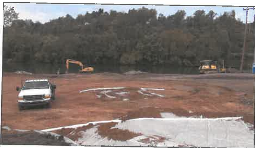
West Virginia DNR New 3 Lane Boat Ramp Construction
